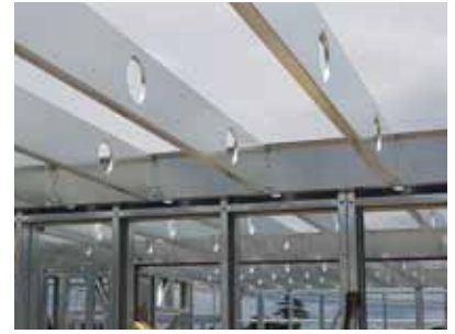
UP TO 7.25 METER SPANS OPENING UP ROOM DESIGN
