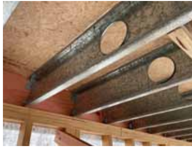
EZYJOIST TO TIMBER CONNECTION
